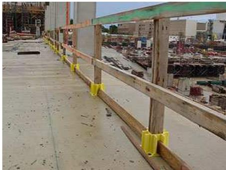
We have added into stock these safety boots. The reusable Safety Boot allows you to quickly construct freestanding railings for stairways, ramps, walkways, balconies and/or roofs. Utilizing job site tools, specified fasteners and construction grade 2x4s, the durable Safety Boot Guardrail System is the most cost effective solution for temporary railings. And, since the Safety Boot requires no bracing, the Safety Boot Guardrail System can remain in place throughout construction, including drywall!
